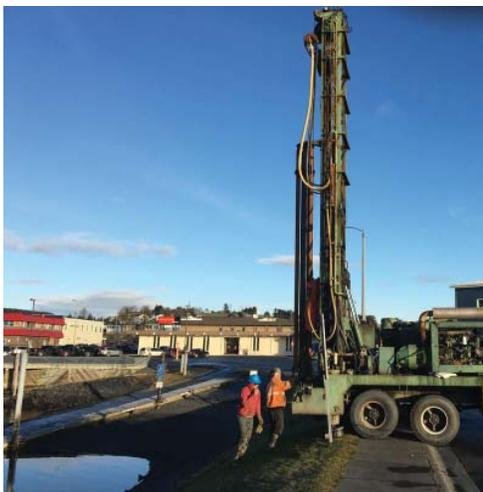
*Mill Bay Drilling boring test holes on the Thelma C site in early December*
