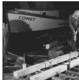
Commercial Marine yard at Lake Union photo: Commercial Marine Construction
